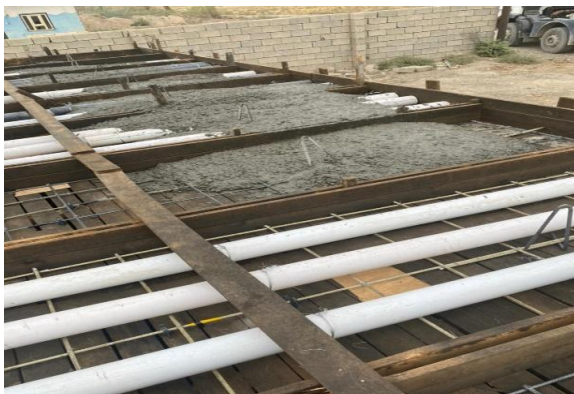
Figure (3) shows casting the concrete for the slabs.
