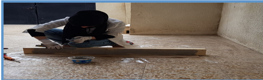
4. Application of jute fibers on the epoxy.
