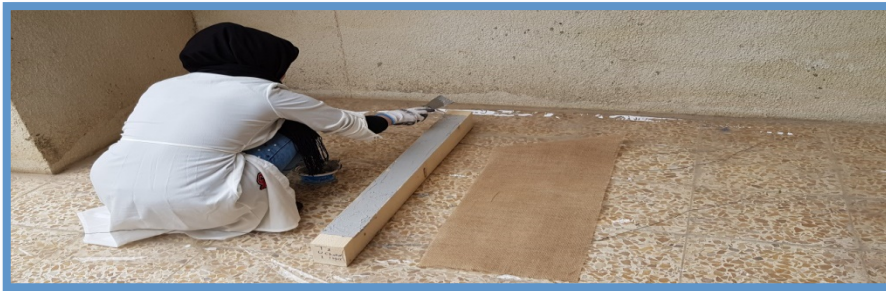
3. Application of epoxy on the beam.
