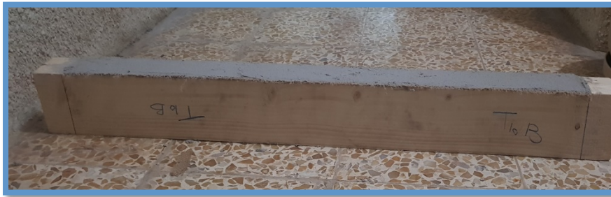
8. Flexural strengthening in three layers.
